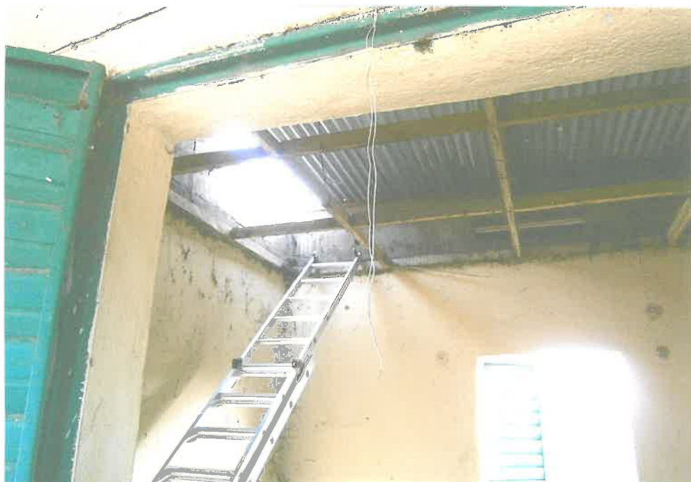
Dachreparat. Geburts- station
